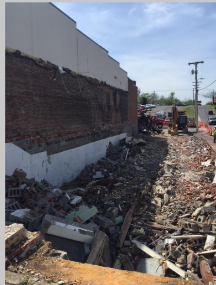
The former Archery Building was demolished on April 19, 2016.
