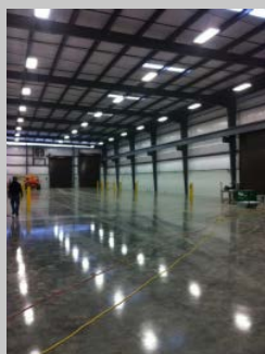
Forestry Equipment of Virginia's 42,000 square foot new addition.
